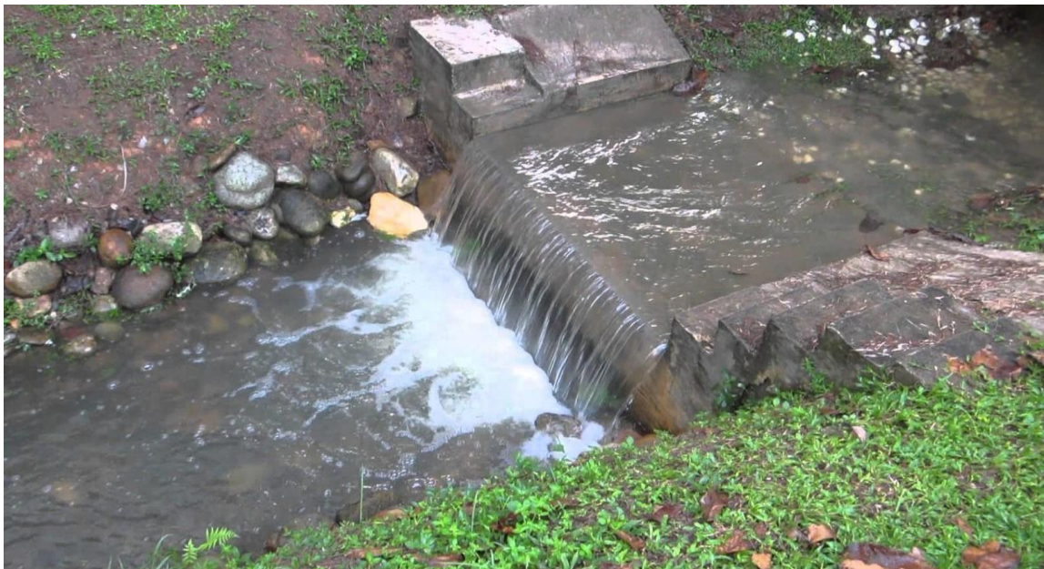
Figure 1.2: Broad-Crested Weir in the Field.
